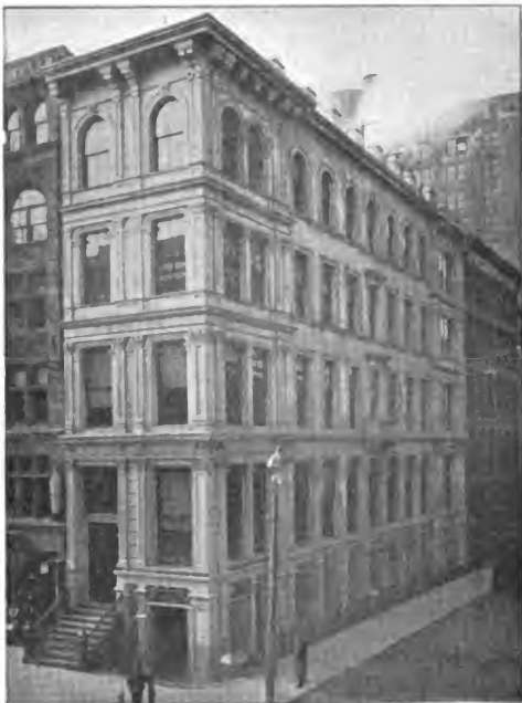
MERCANTILE NATIONAL BANK, BROADWAY AND DEY STREET.
